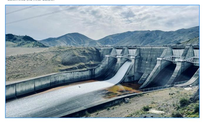
The spillway comprises four spillway gates and two sluice gates. The runoff down to the river is 450 metres in length with a huge block of concrete – an energy dissipater – at the end of the spillway to reduce the power of the water flow into the river. With that, our visit to Benmore finished and there was just about time for a sprint back to the airport in Twizel for a flight to Melbourne, Australia.
