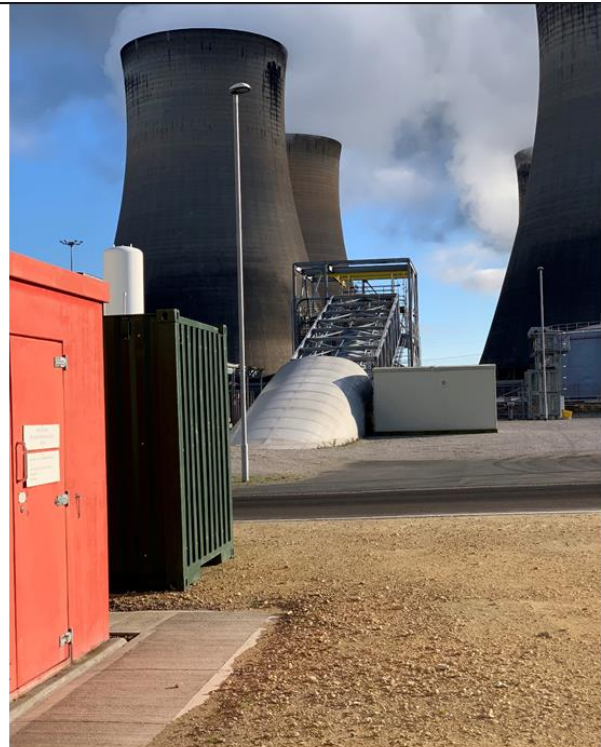
The covered conveyor belt emerges from the ground transporting pellets away from the biomass domes
